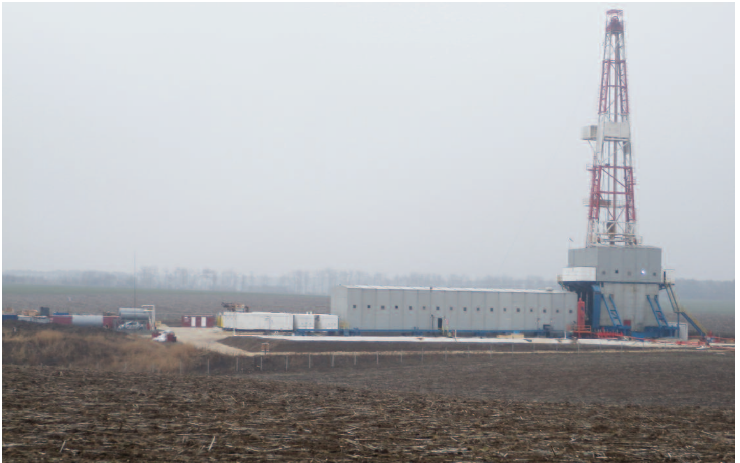
Caption: Drilling pad in Bulgaria. Each pad requires almost 4 hectares to install all the necessary equipment for extraction.
